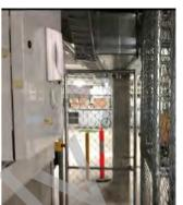
**D2 MACHINE ENCLOSURE:** Machine enclosure has many open penetrations that need permanent fixings to cover up these areas.
