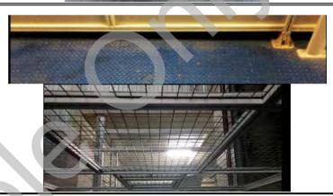
**D7 MACHINE ENCLOSURE:** Machine enclosure floor leaks oil and there are penetrations that need filling.
