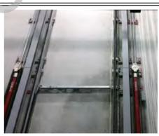
**D4 PLATFORM CLEARANCE:** Platform clearances are too small or too large and should be no less than 25mm and no more than 50mm. These clearances should be corrected.
