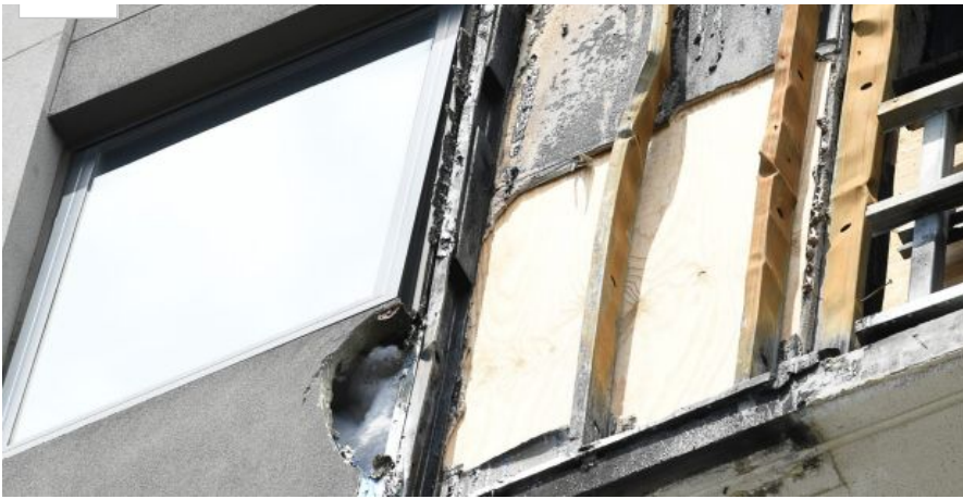
A fire caused major damage to the Brunswick building earlier this year. Photo: Justin McManus
