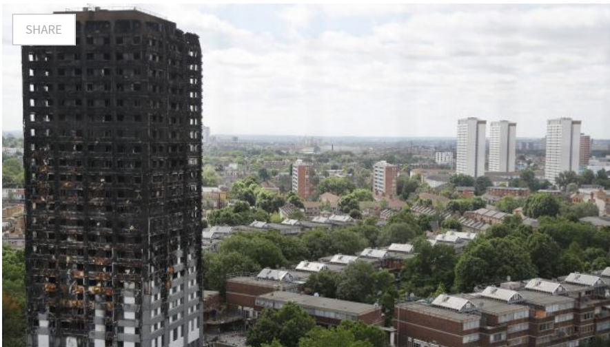
Some of the cladding on the Brunswick apartments is the same as that which was used on London's Grenfell Tower Photo: AP
