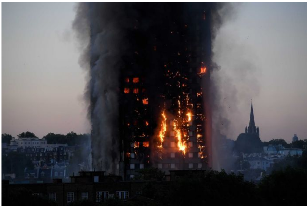
PHOTO: The Grenfell Tower fire in London was the catalyst for a statewide Victorian audit for combustible cladding. (Reuters: Toby Melville)
