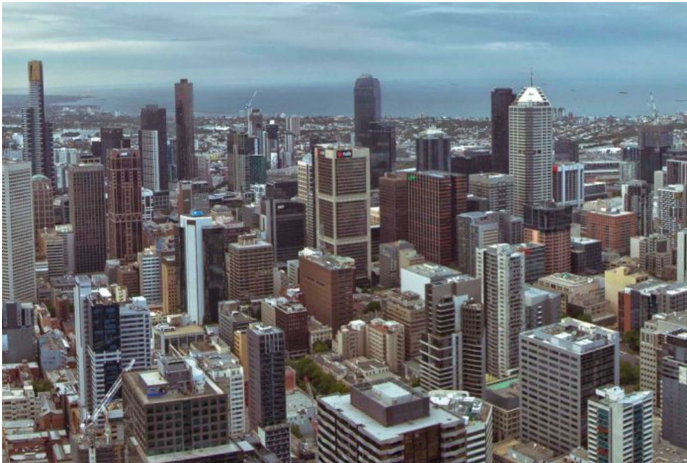
PHOTO: Dangerous, combustible cladding could be a risk on 1,400 Victorian buildings. (ABC News: Margaret Burin )
