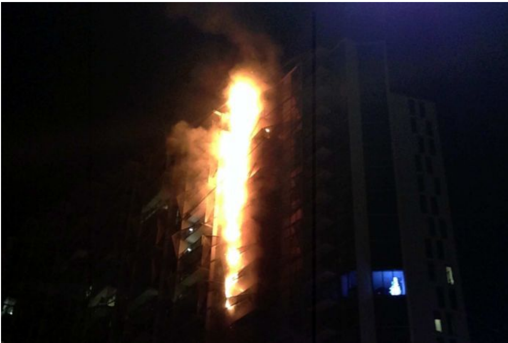
PHOTO: The Lacrosse apartment building in Melbourne's Docklands caught on fire in November, 2014. (Audience submitted: Wade Savage)
