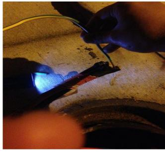
Roscon personnel conducting the required testing by making a circuit to the switchboard with new cabling. Roscon had cordoned off the area to the public for OH&S, and using vehicles for temporary lighting.
