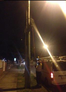
This photo illustrates the United Energy staff connecting the fuse back into the power pole.
