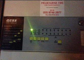
Roscon also isolated the fire indicator panel (FIP) prior to restoring power to ensure no false alarms were sent to the MFB resulting in a call out.
