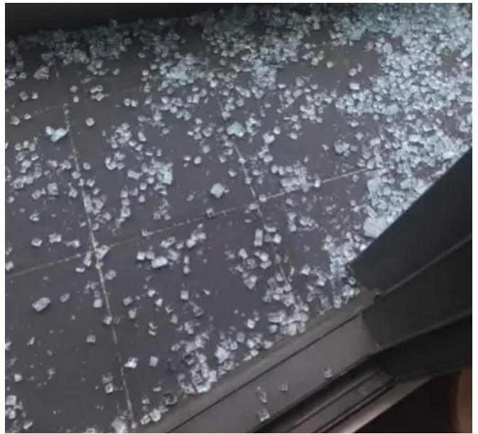
Glass fell onto the balcony of the apartment below.
