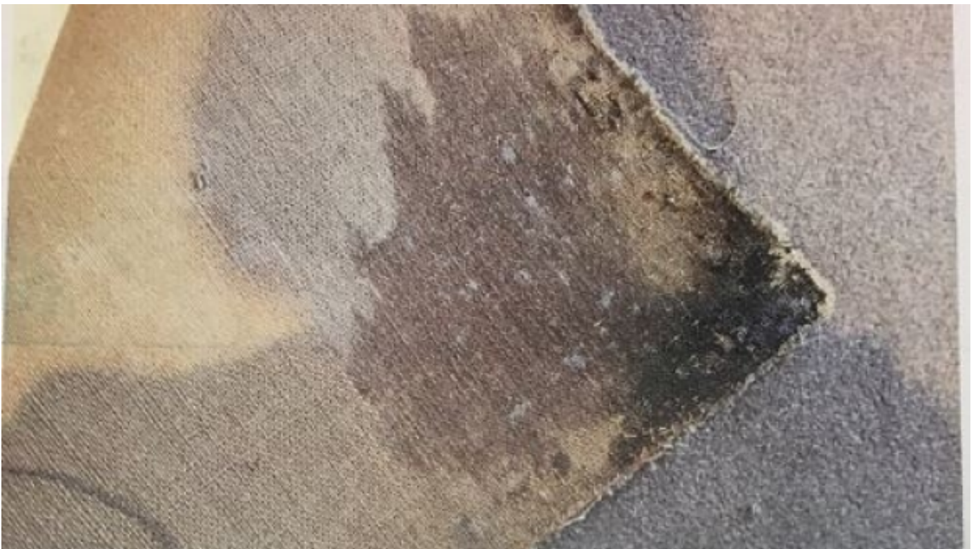
Mould and water damage to the carpet in Julie Gaffney's Abbotsford apartment. Photo: Supplied
