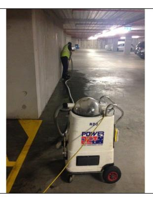
Extraction of the black water (sewage/grease) commenced and the area was blocked off.
