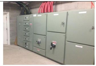
After the black water extraction commenced and the area was blocked off. Roscon also commenced trouble shooting the commercial tenancies power outage. Albert provided access into the main electrical distribution rooms, all circuits were tested and one was tripped which was reset and power returned to the commercial tenancies.
