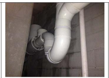
This is the pipe which was blocked and caused the sewage to back flow into the grease trap and subsequently overflow the grease trap.
