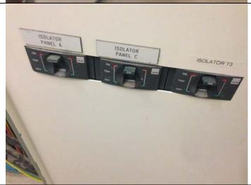
After the black water extraction commenced and the area was blocked off. Roscon also commenced trouble shooting the commercial tenancies power outage. Albert provided access into the main electrical distribution rooms, all circuits were tested and one was tripped which was reset and power returned to the commercial tenancies.
