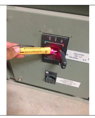
After the black water extraction commenced and the area was blocked off. Roscon also commenced trouble shooting the commercial tenancies power outage. John provided access into the main electrical distribution rooms, all circuits were tested and one was tripped which was reset and power returned to the commercial tenancies.
