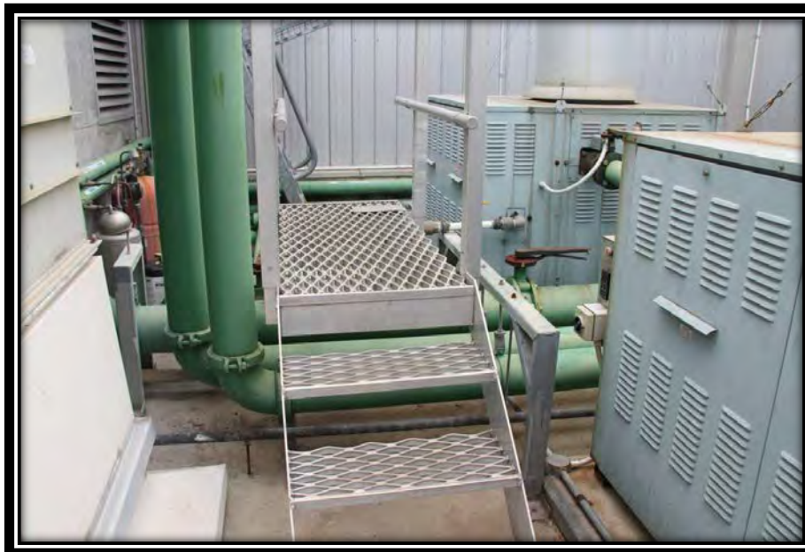
Condenser water pipes cat way example.
